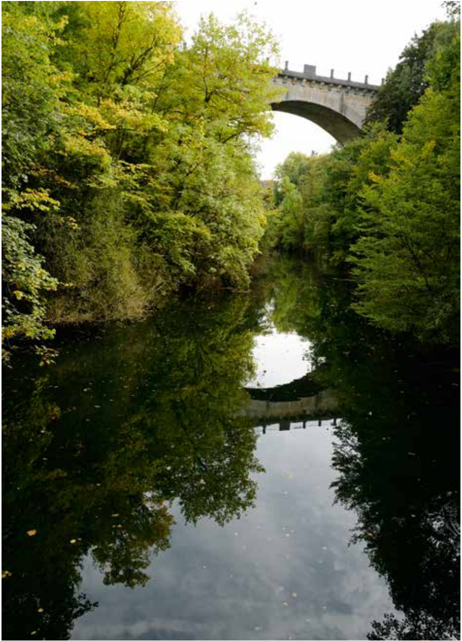
Grand Pont on the Orbe River, Orbe, Switzerland
